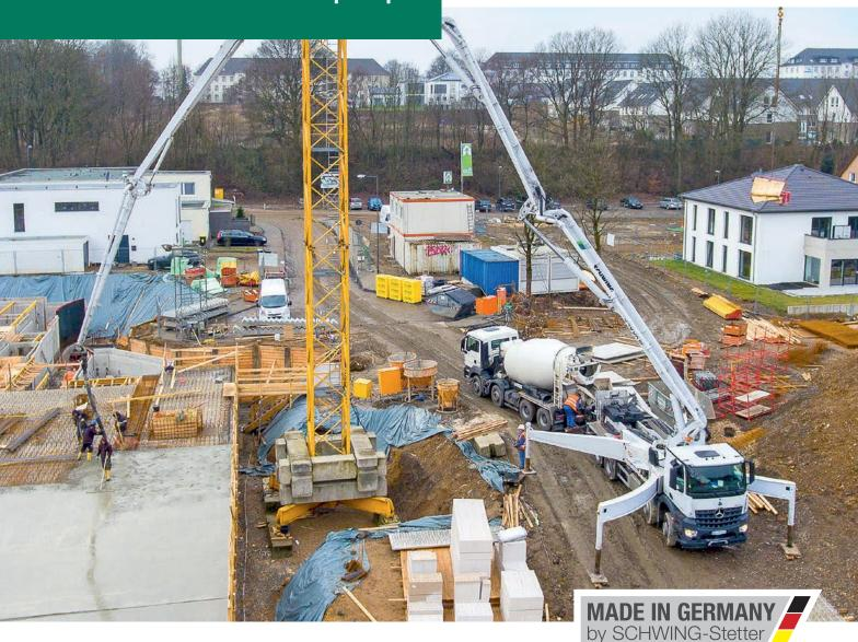
Vertical reach 42.30 m Concrete output max. 162 m³/h Pressure on concrete max. 85 bar
